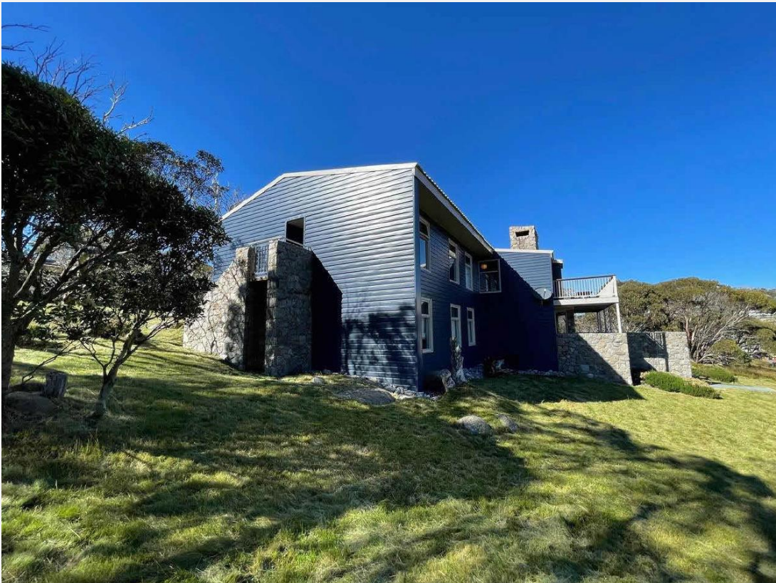
Figure 4 | View of Lodge from the north
